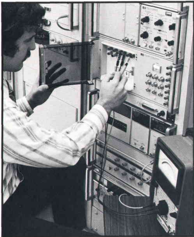
Fig. 2. High voltages in 9550 Systems appear behind this interlocked safety door. Hardware and software interlocks are provided.
